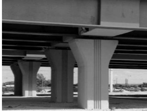
Fig. (1.15): Pier foundations.
