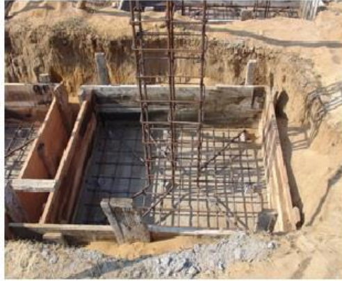
Isolated RCC Footing
