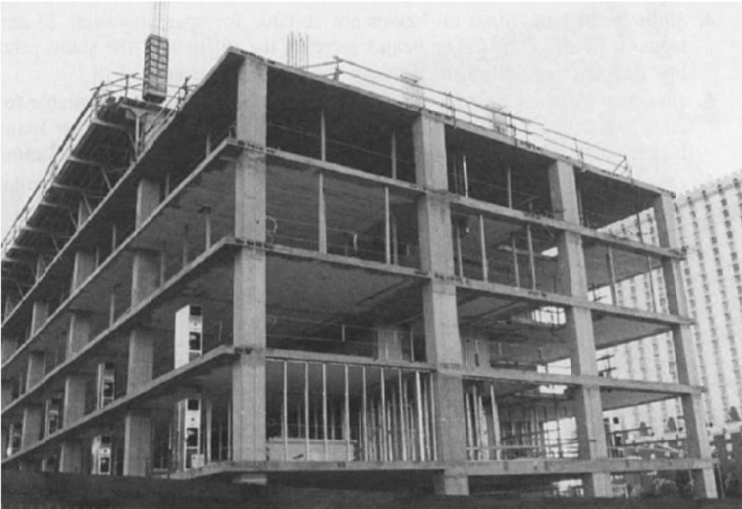
Flat-plate floor system.
