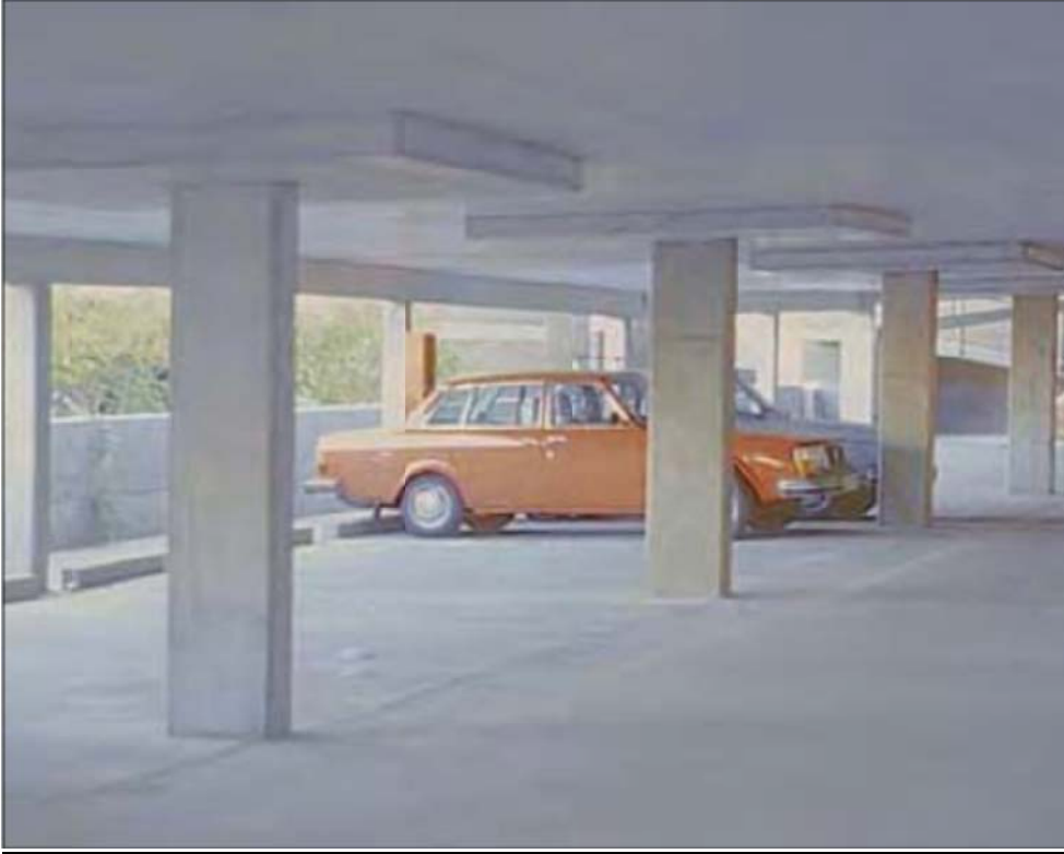
Flat Slab floor system
