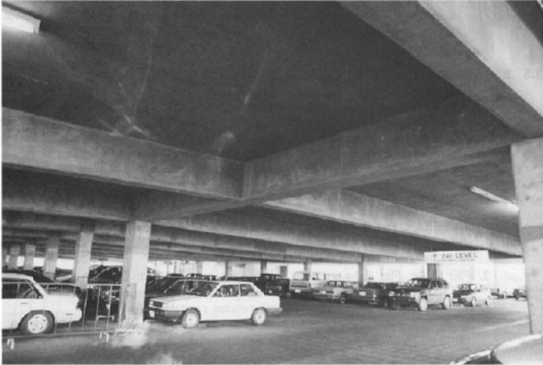
Slab on beams.
